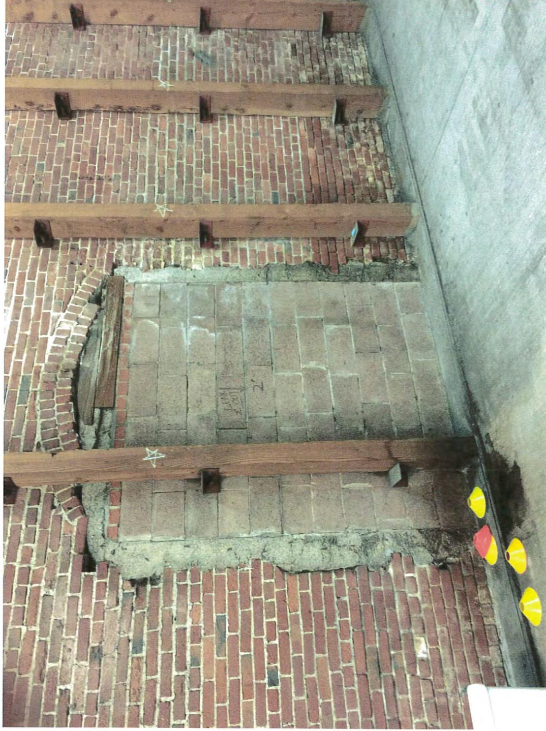
Opening of Building "B" showing the area that was original. These area's were filled in with block and brick and will be restored per drawings.
