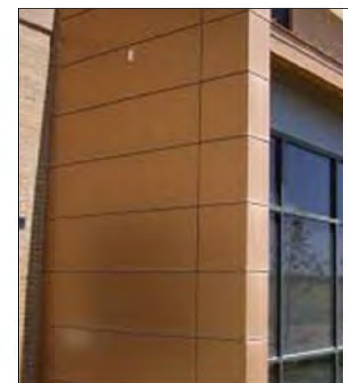
3 PANELIZED BUILDING CLADDING SYSTEM
