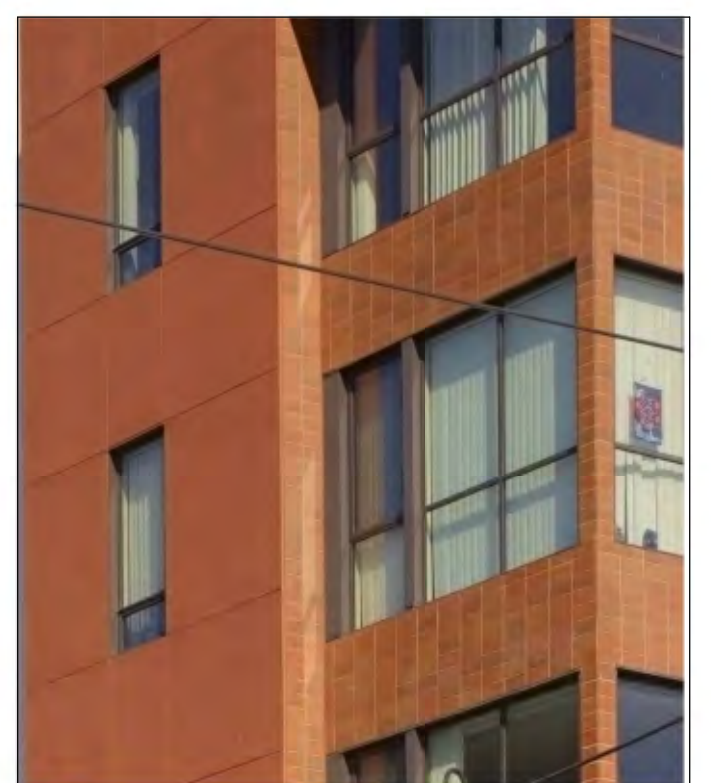
5 SELF RECESSED ALUMINUM WINDOW SYSTEM - DARK BRONZE WITH CLEAR AND OPAQUE GLAZING - ON STREET FACADES
