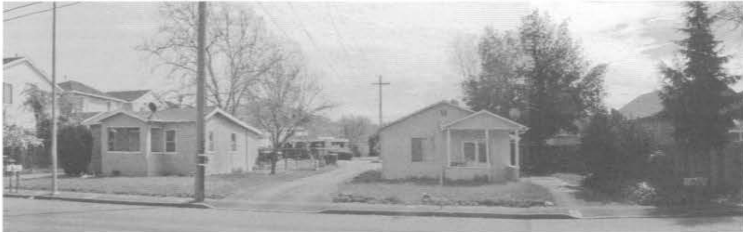
1-FRONT OF PROPERTY LOOKING SOUTH
