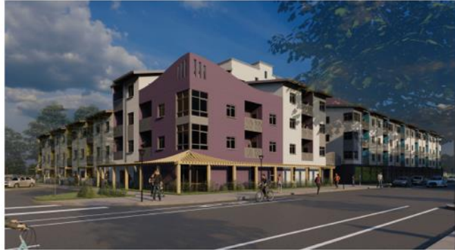
MAIN BUILDING CORNER
