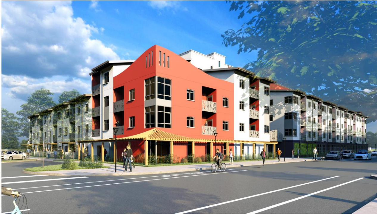
MAIN BUILDING CORNER
