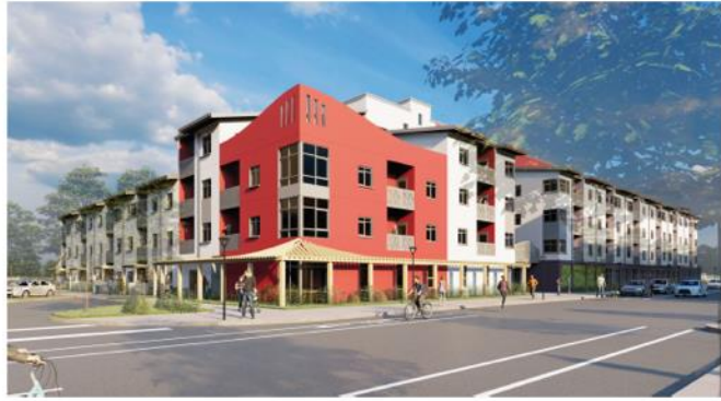
MAIN BUILDING CORNER
