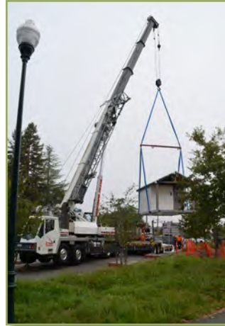
Keiser Bathroom Install
