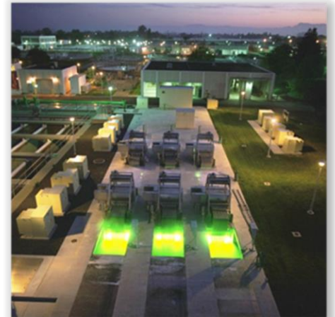
Laguna Treatment Plant
