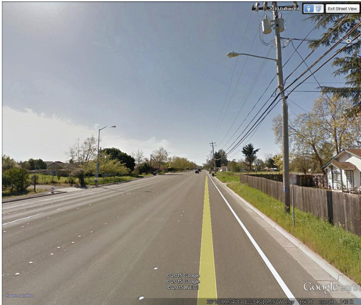
Phase 1 looking south (Completed)
