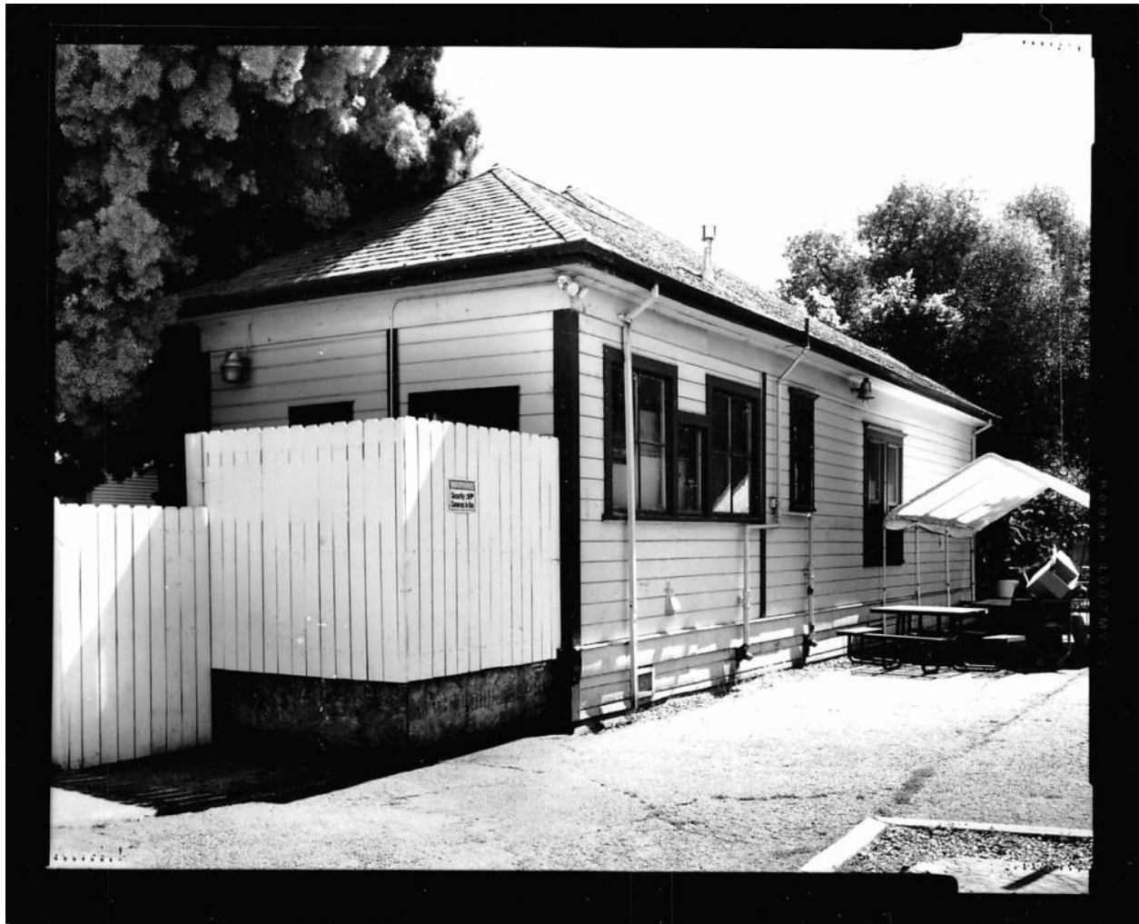
520 Morgan Street - Photo #6 - EXTERIOR, OVERVIEW OF NORTH (SECONDARY) FAÇADE AND PARTIAL EAST (REAR) FAÇADE, VIEW TO SOUTHWEST.
