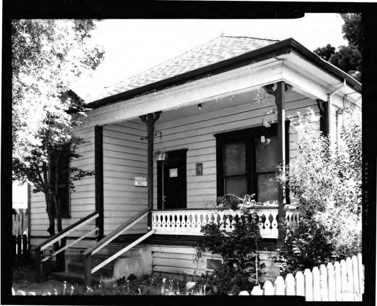
520 Morgan Street - Photo #1 - EXTERIOR, OVERVIEW OF WEST (PRIMARY) FAÇADE, VIEW TO NORTH.
