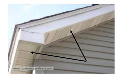
Vent requirements – there shall be modifications to structural vent openings as to resist building ignition through the intrusion of burning embers and flames through the ventilation openings. There are specific criteria that must be met for compliance with these requirements.
