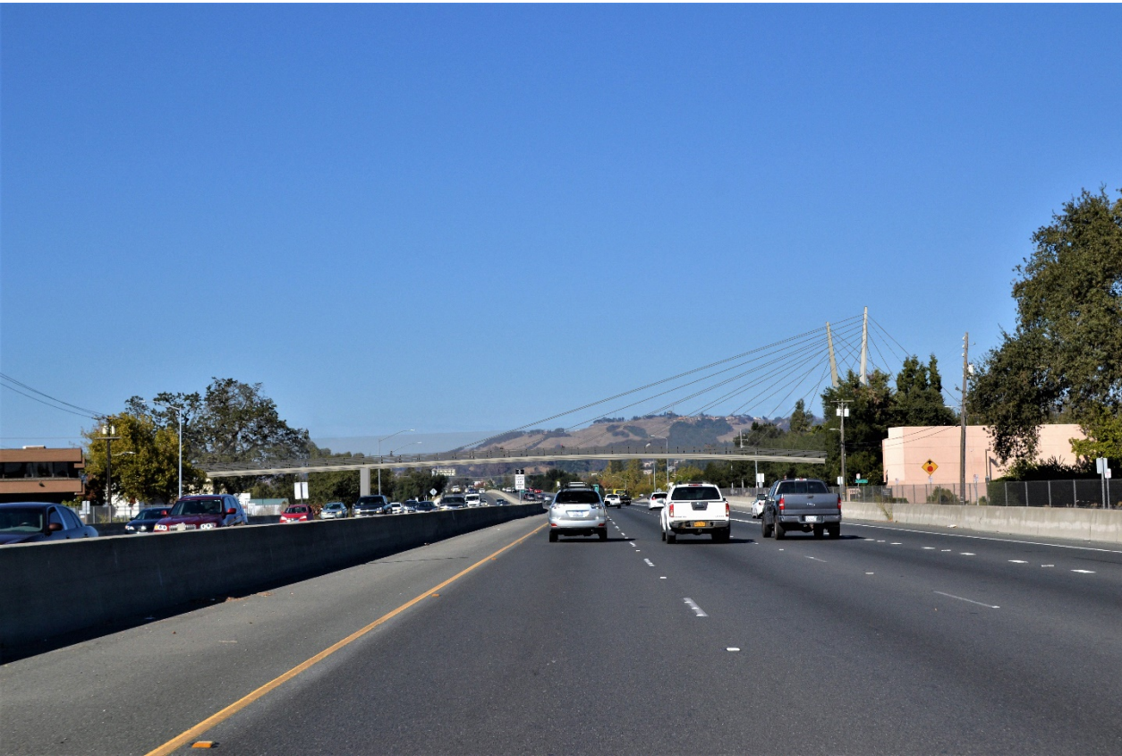
View from US 101 northbound
