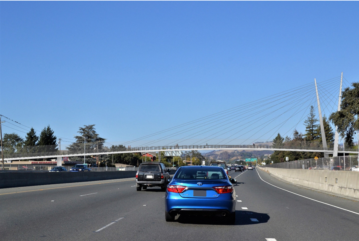
View from US 101 northbound
