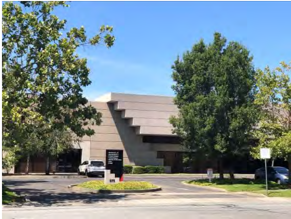
Photo #13 View of the multi-tenant warehouse building (975 Corporate Center Parkway) located to the adjoining west of the site.
