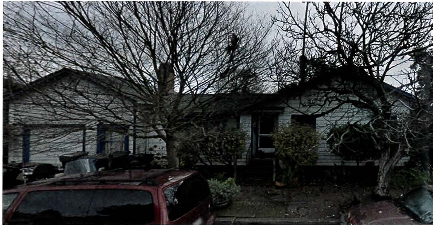
Original West 6th Street Elevation
