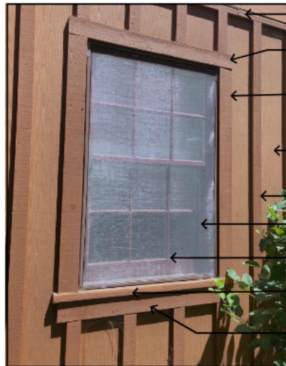
WINDOW/DOOR TRIM, SIDING DETAIL
