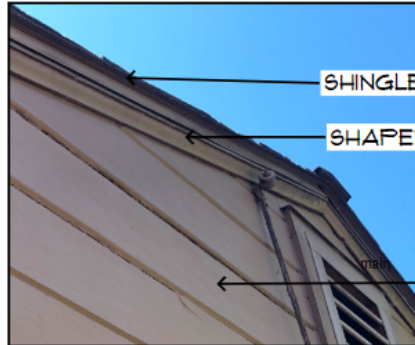
RAKE WALL DETAIL
