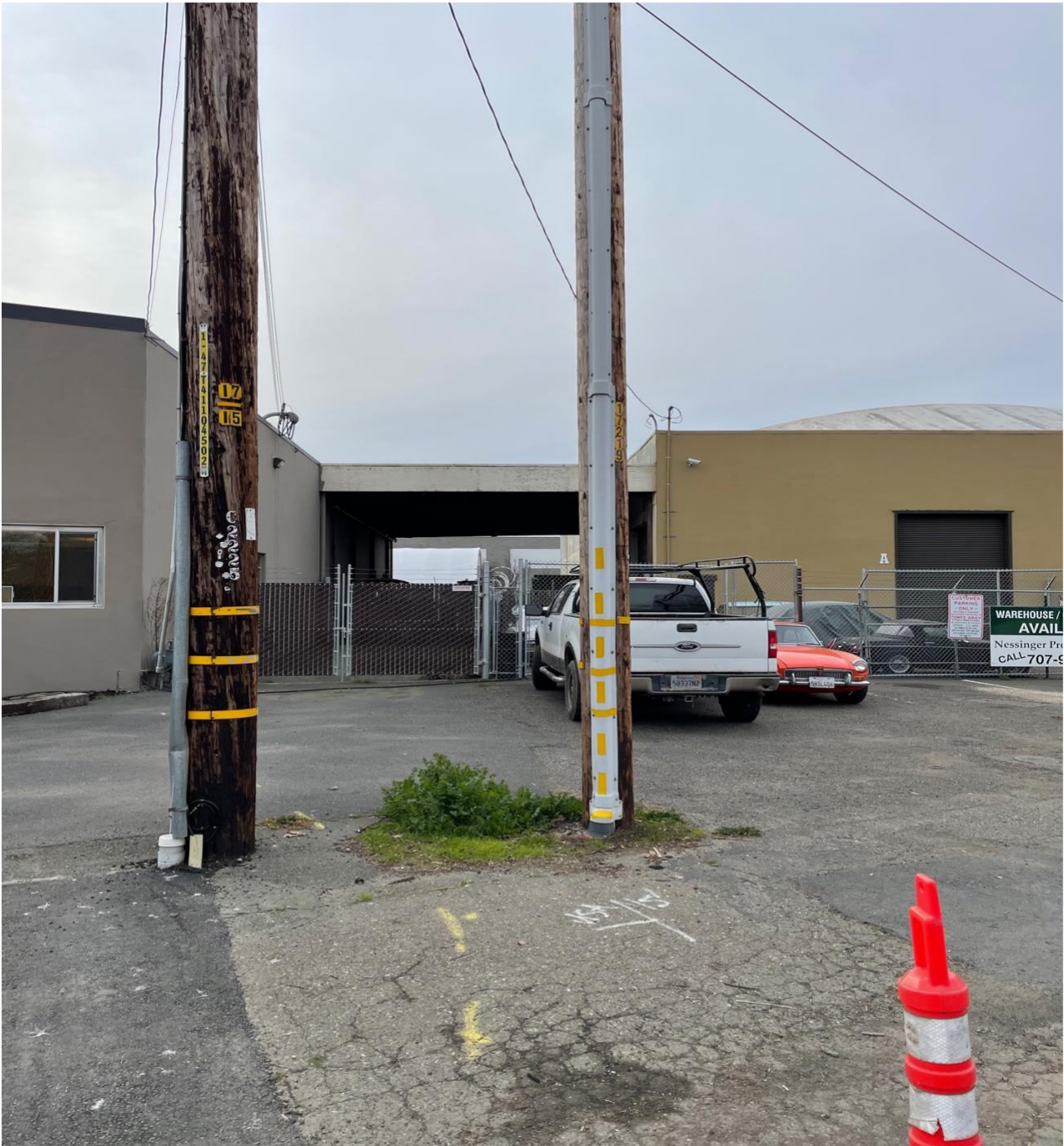
Current Entry Gate
