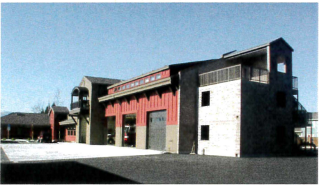
The City of Sonoma Fire Headquarters, Sonoma, CA (top to bottom) Public Entry, Fire Trucks & Apparatus Bays, Training Tower (RossDrulisCusenbery Architecture, Inc.)
