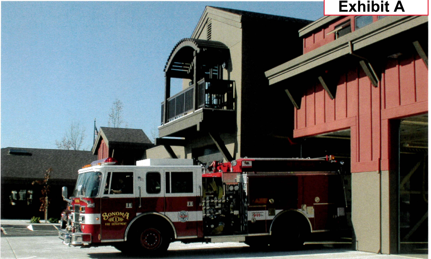
Sonoma Fire Department Headquarters & Training Facility (Architects: RossDrulisCusenbery Architecture, Inc.)
