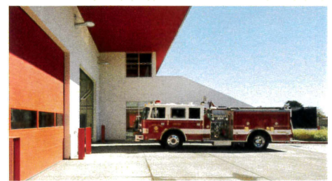
Cherryland Fire Station & Future EMS Health Portal Alameda County, CA (RossDrulisCusenbery Architecture, Inc.)
