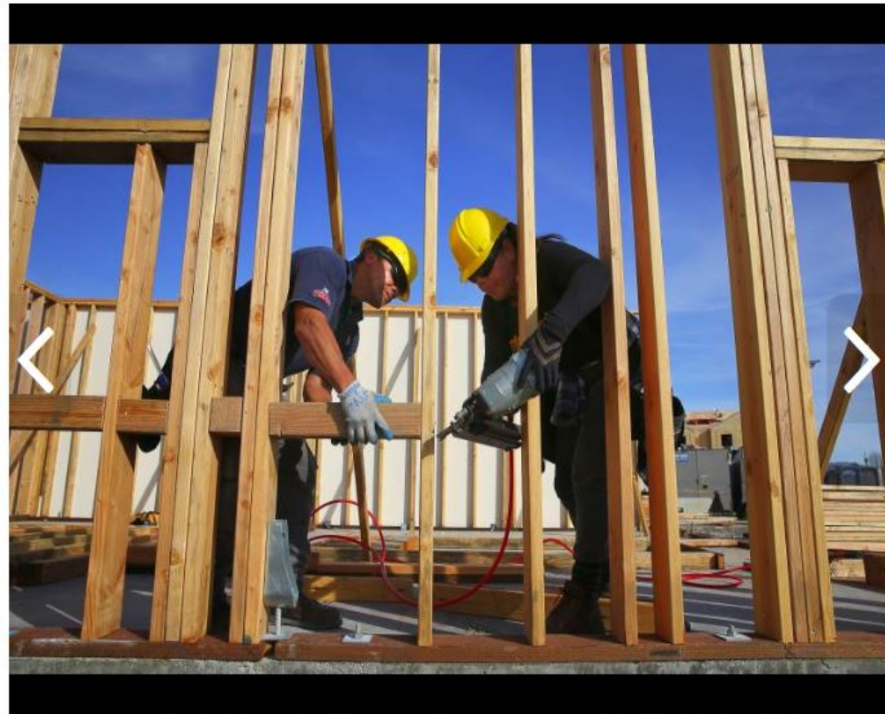
(1 of 3) Owner/builders Jose Castro, left, and his wife, Ana Espinoza, work on a new residential home at Catalina Homes, by Burbank Housing, in Santa Rosa on Monday, February 22, 2016. (Christopher Chung/ The Press Democrat)
