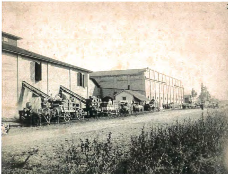
View of the west elevation of the DeTurk Winery, where bottles are being loaded onto carts, ca.1880. A gabled roof office building is located in front of the brick winery. Photo courtesy of the Healdsburg Wine Library, Healdsburg, CA.
