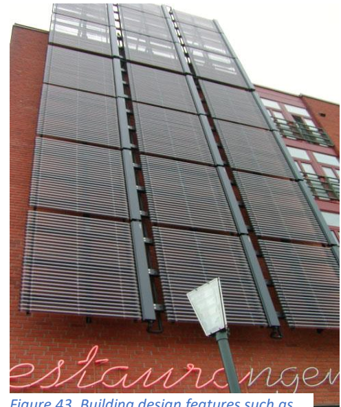
Figure 43. Building design features such as screens help improve environmental quality
