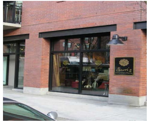
Figure 38. Example of a detailed façade at street level.
