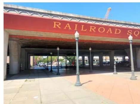
Figure 17. Underpasses should include special lighting and artwork.
