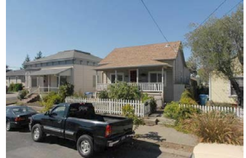
Figure 39. Existing residences in the West End Preservation District
