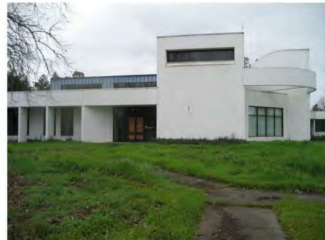
Photo 2: Southwestern-facing view of the northeastern-most commercial building referred to as the former Sonoma County Water Agency Operations & Maintenance Building.
