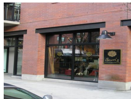
Figure 38. Example of a detailed façade at street level.
