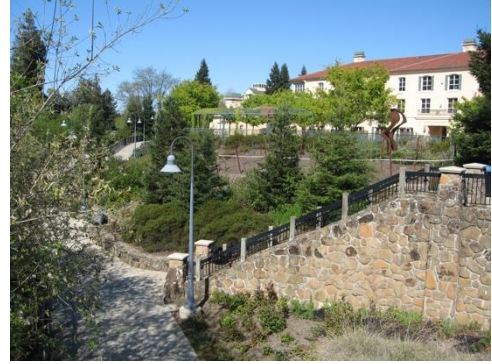
Figure 27. Creekside oriented development - the Hyatt Vineyard Creek Hotel adjacent to Santa Rosa Creek
