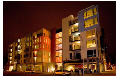
Figure 29. Example of a well-designed multi-tenant, pedestrian-oriented development.
