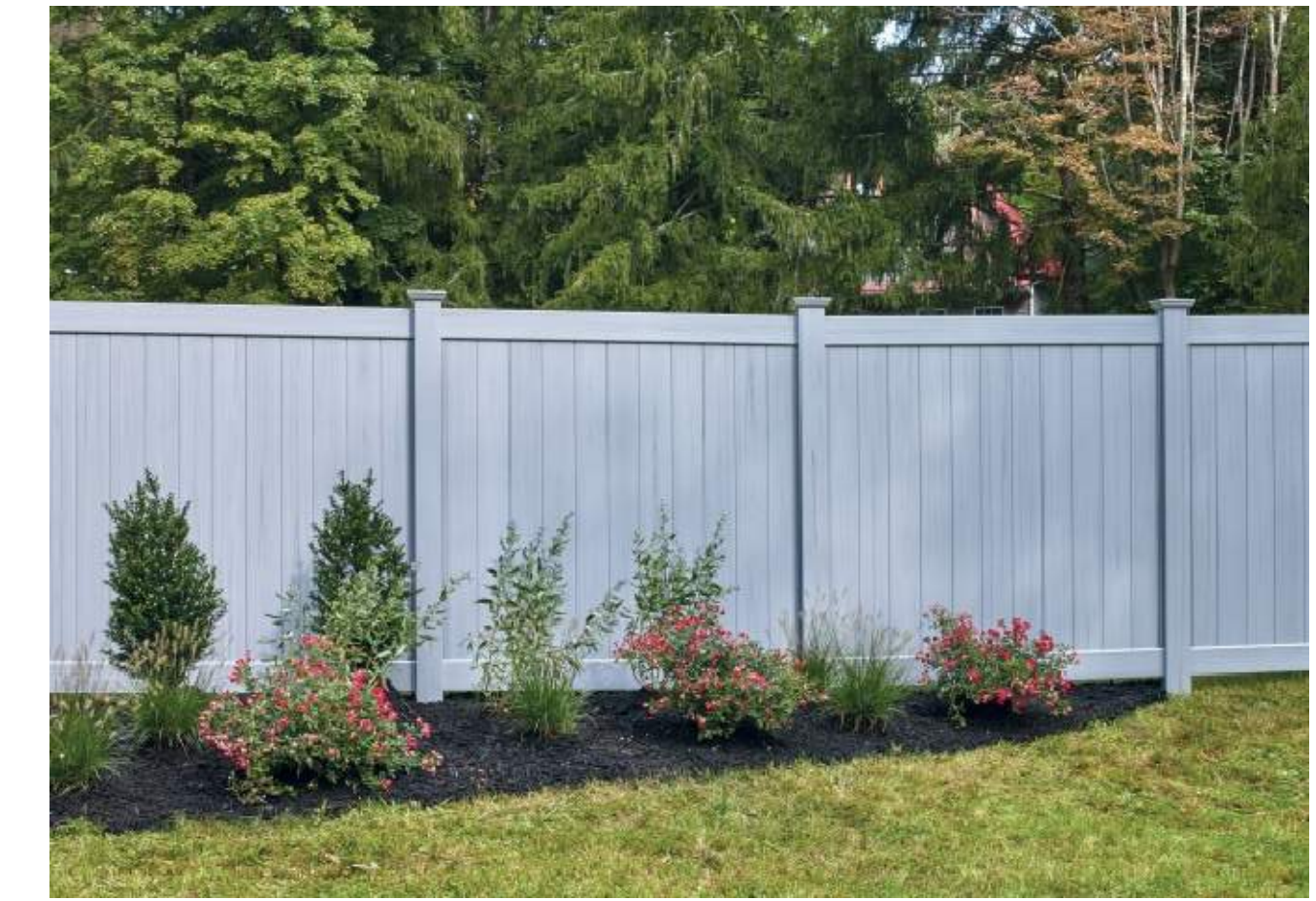
6'-0" NOMINAL HEIGHT WOOD OR VINYL PERIMETER FENCING
