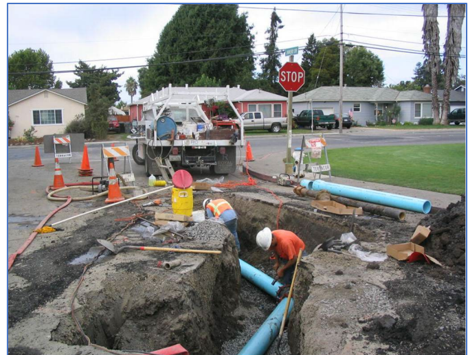
Installation of Water Distribution Main
