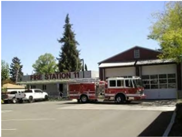
Figure 76: Santa Rosa Fire Department Station 11 550 Lewis Road
