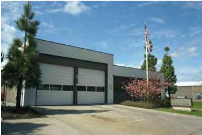
Figure 68: Santa Rosa Fire Department Station 2 65 Stony Point Road
