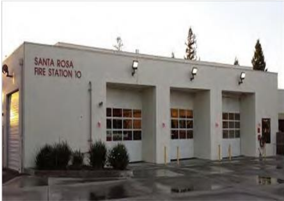
Figure 75: Santa Rosa Fire Department Station 10 1345 Corporate Center Parkway
