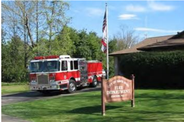
Figure 73: Santa Rosa Fire Department Station 7 6590 Stone Bridge Road
