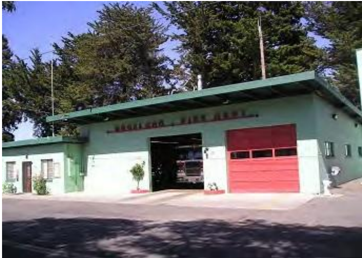
Figure 74: Santa Rosa Fire Department Station 8 830 Burbank Avenue
