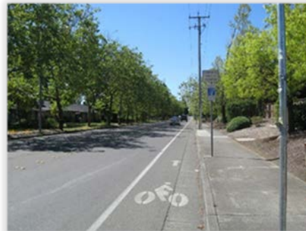
Miles of Road 493 Center Line Miles 2,097 Lane Miles
