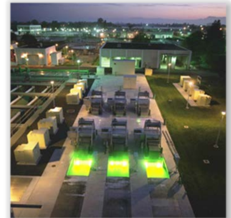
Laguna Treatment Plant
