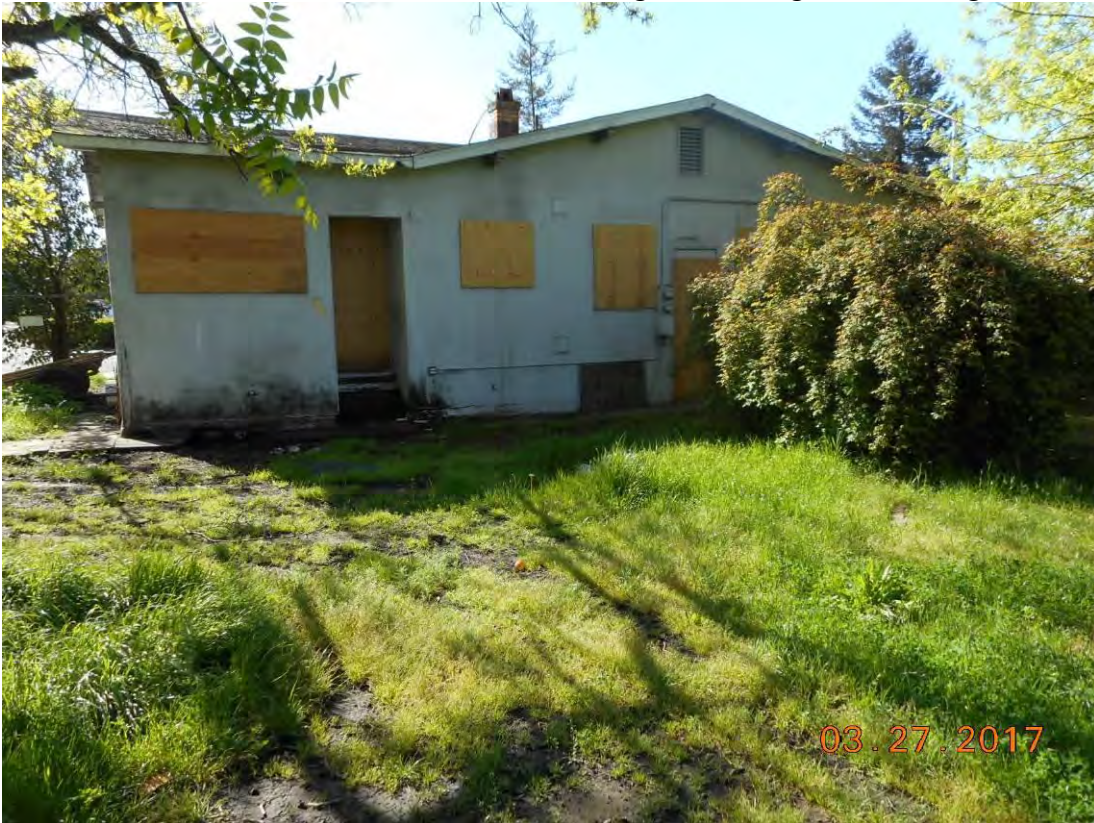
Figure 3. Abandon residence on the proposed project site.
