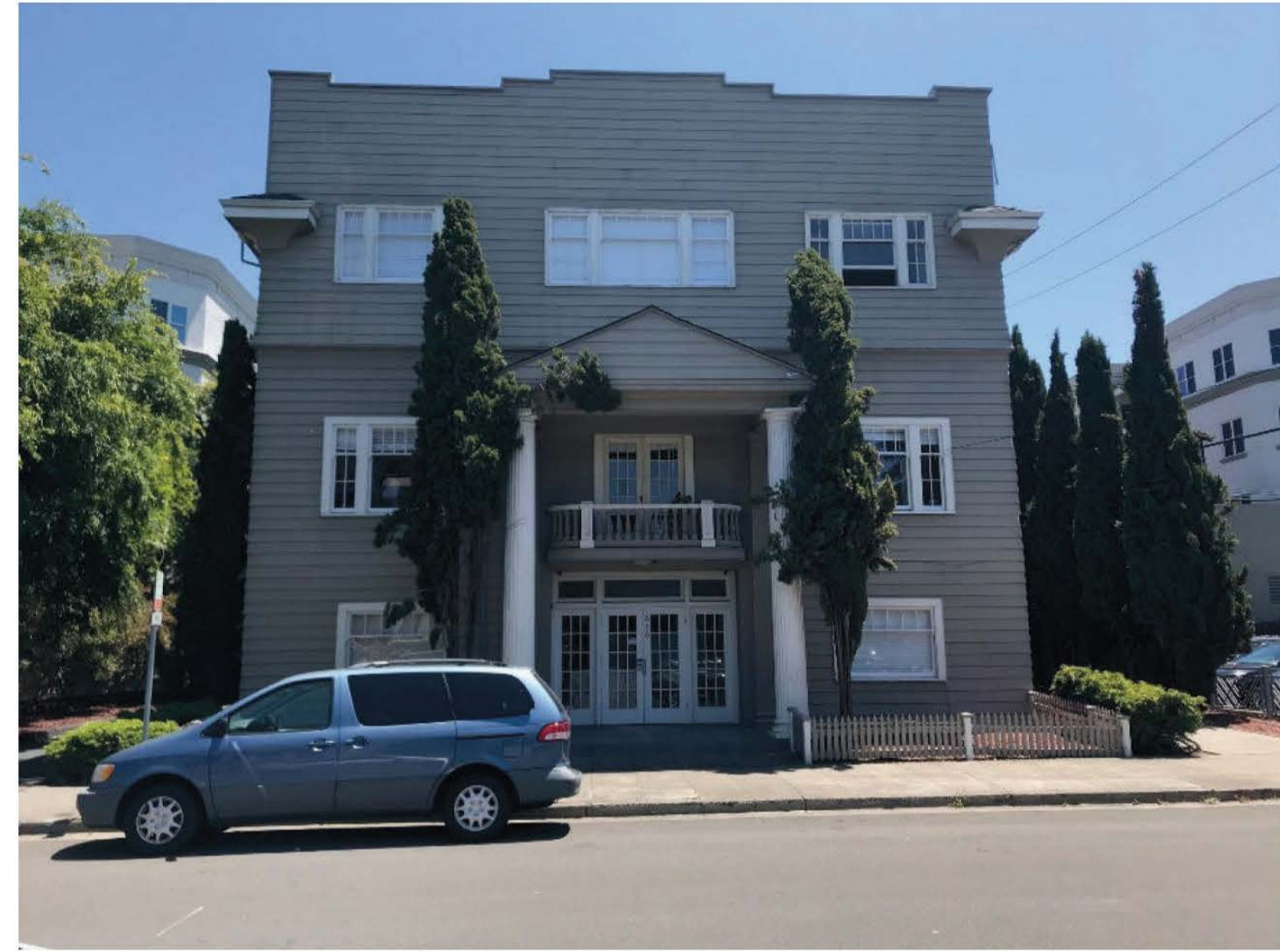
616 B Street - 11 Units
