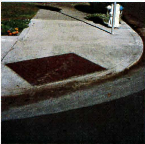
ADA access ramp treatment in Railroad Square district.
