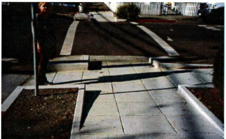
Unique treatment of ADA access ramp with historic garden sidewalk.
