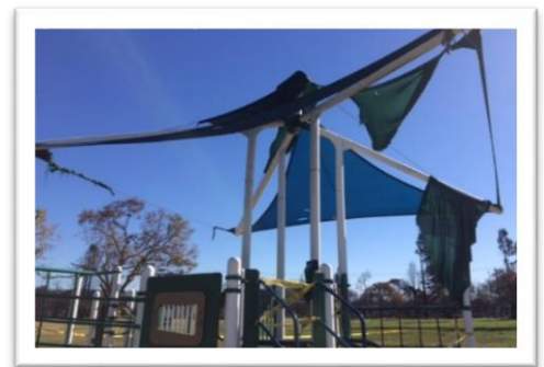
Coffey Neighborhood Park after Tubbs Fire
