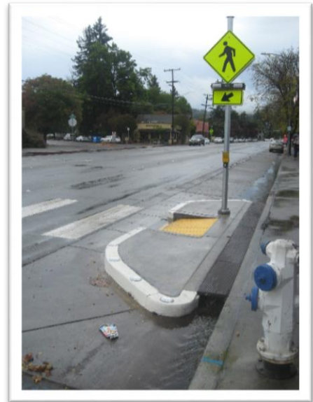
Alderbrook Drive and 4th Street crossing treatment
