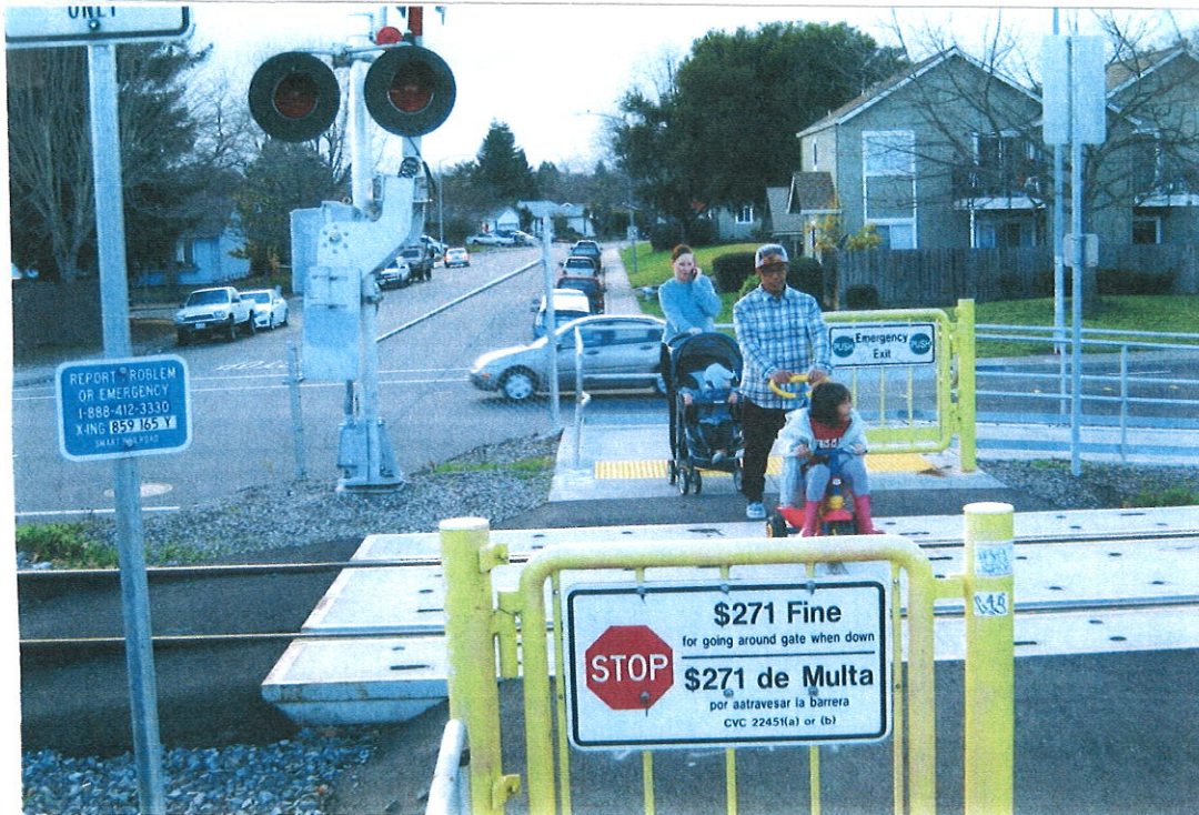
Pedestrian-Bicycle Crossing at Copland Creek Trail (within ½ mile of an Elementary School -- 1/10 /16)
