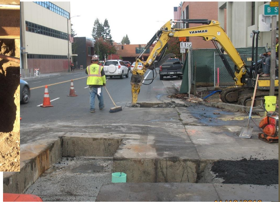
Connecting utilities under Third Street
