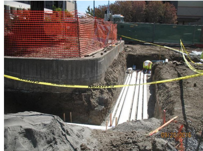
Plumbing for future fountain
