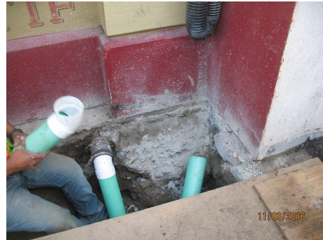
Adjacent property connections
