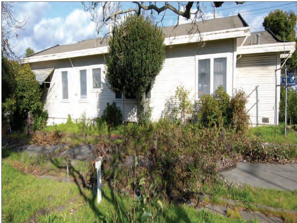
Photo 10. West façade, looking northeast.
