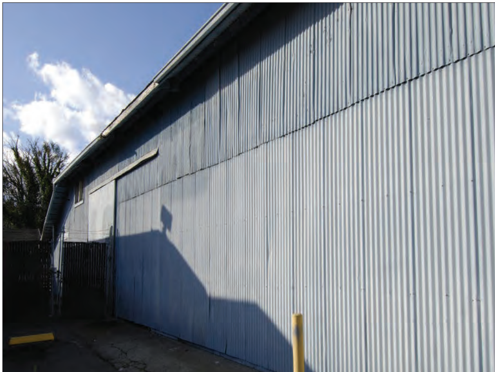
Photo 22. South façade with another sliding barn door.
