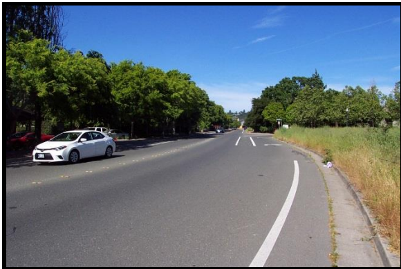
View Northeast Along Kawana Springs Road
