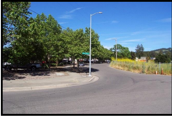
View East From East Boundary Toward Kawana Terrace
