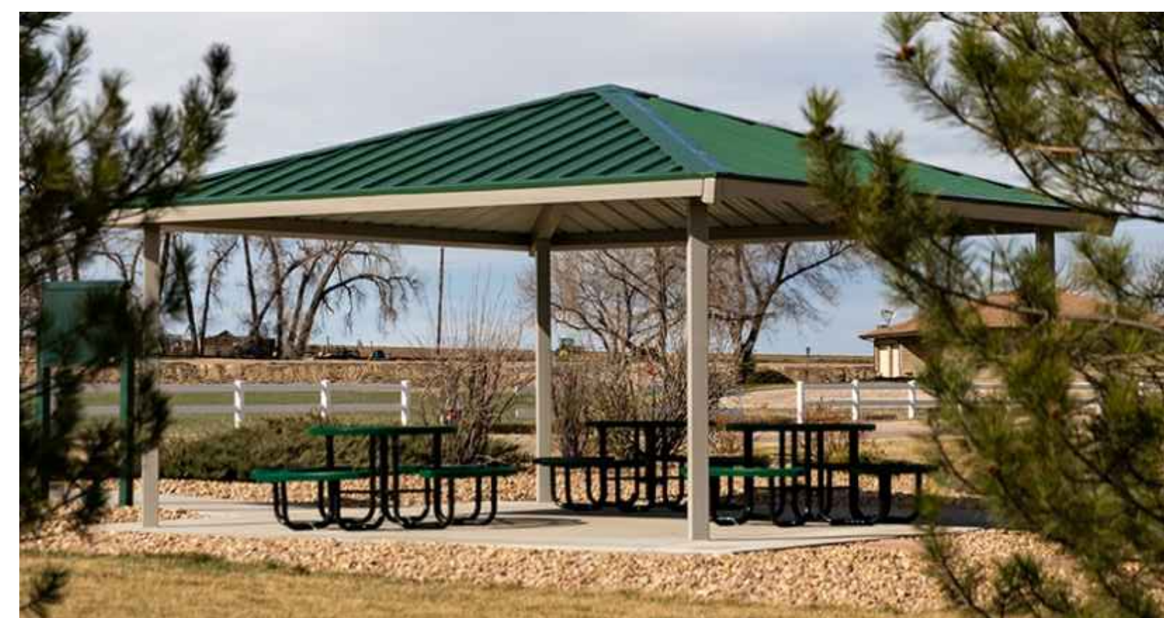
OVERHEAD SHADE STRUCTURE
