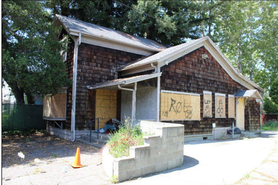
Photo 1: North (front) and east side facade
