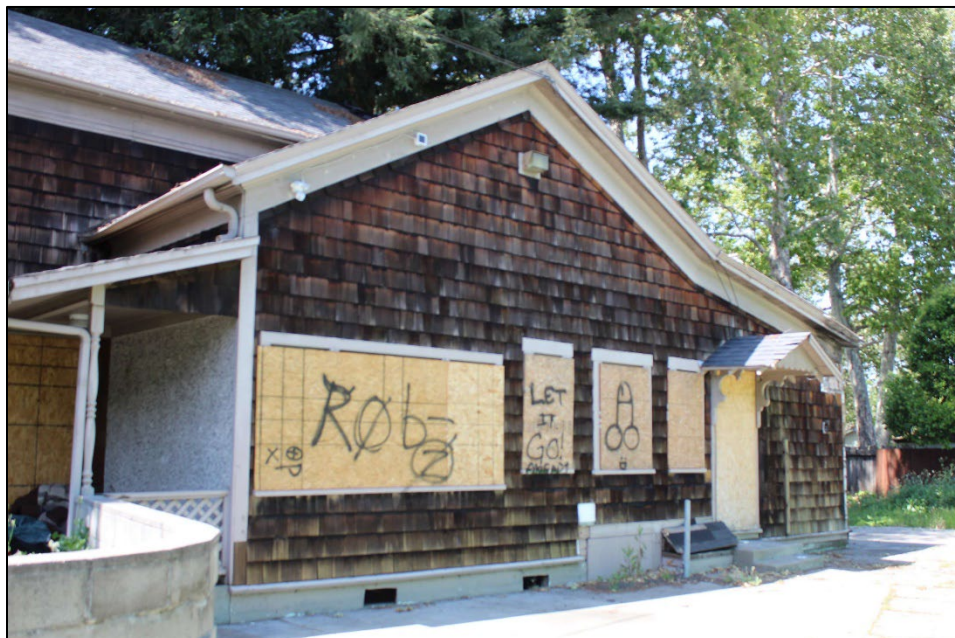
Photo 5: East side façade, looking NW
