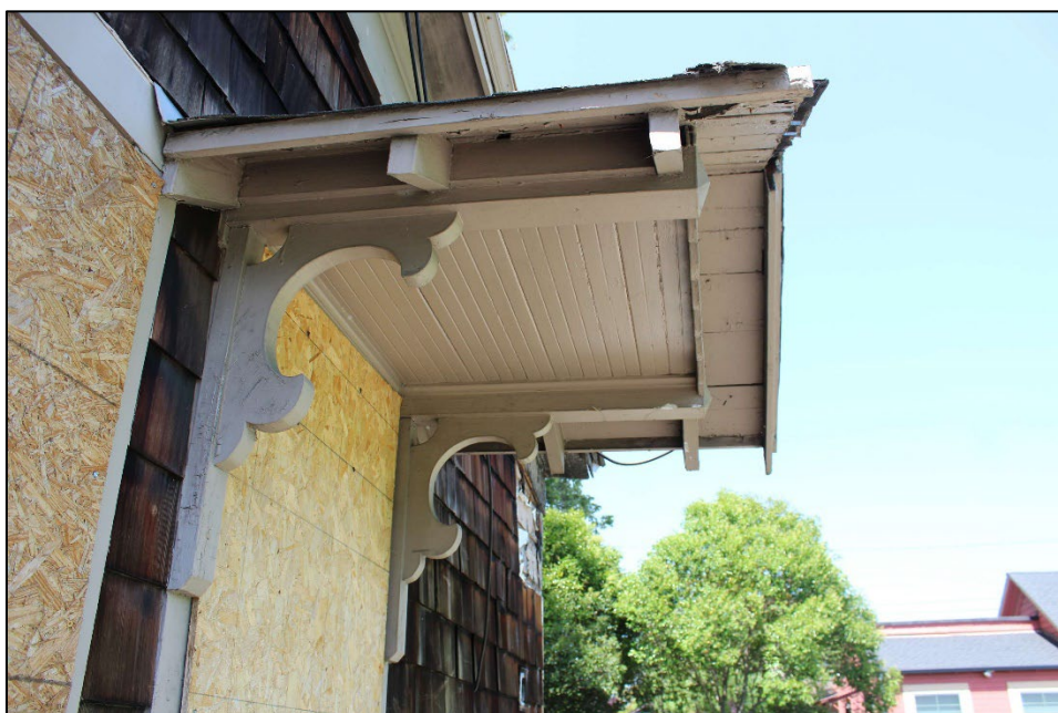
Photo 6: Gable detail, east side facade
