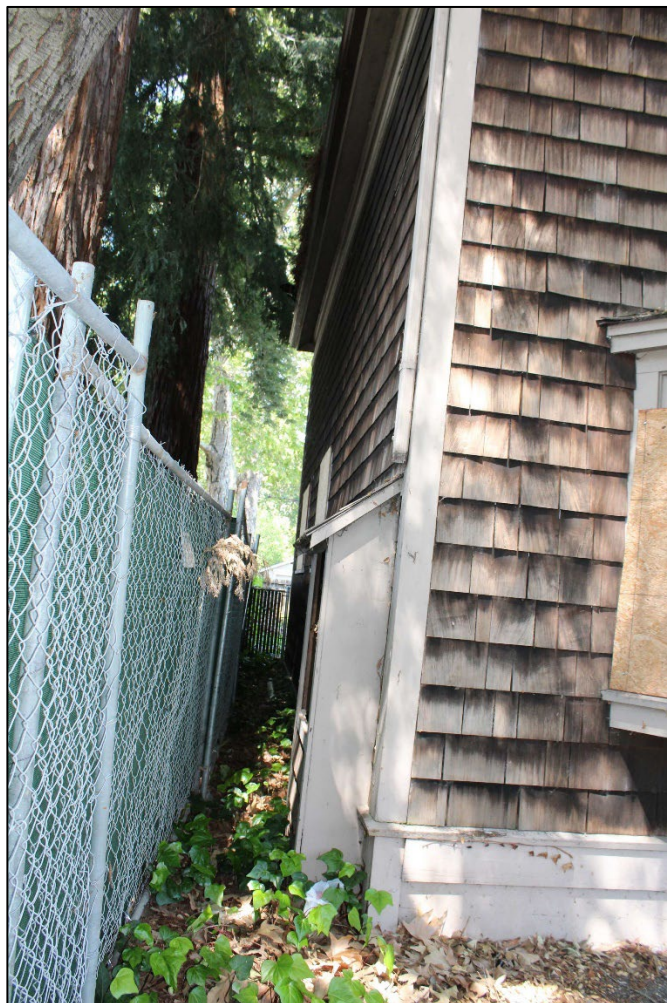
Photo 9: West side façade, looking north
