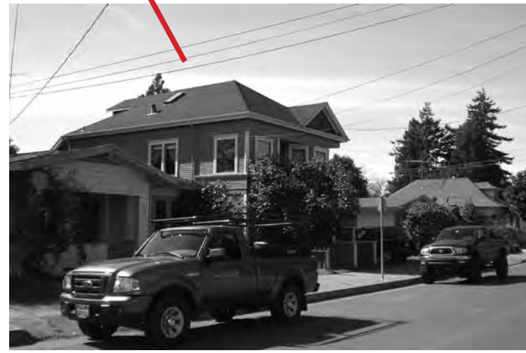
716 TUPPER ST ACROSS THE STREET
