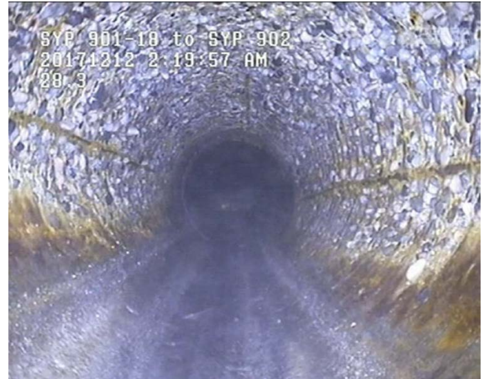
28' In from Inlet Vault
