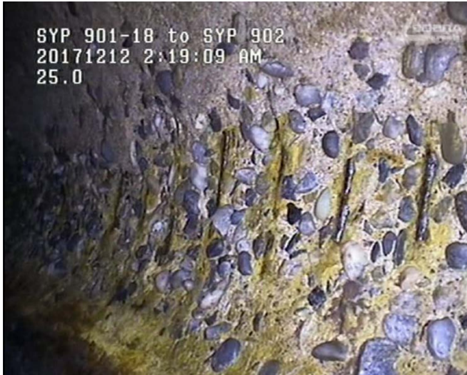
25' In from Inlet Vault
