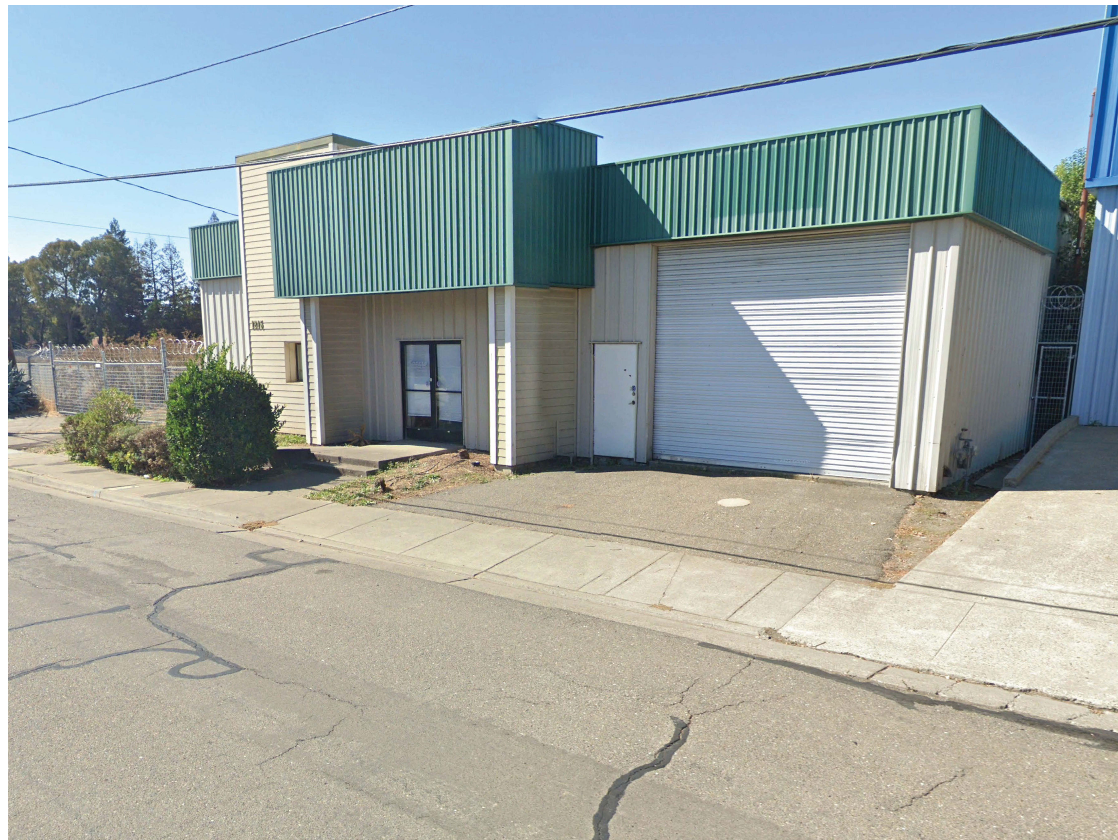
VIEW FROM NORTH EAST
