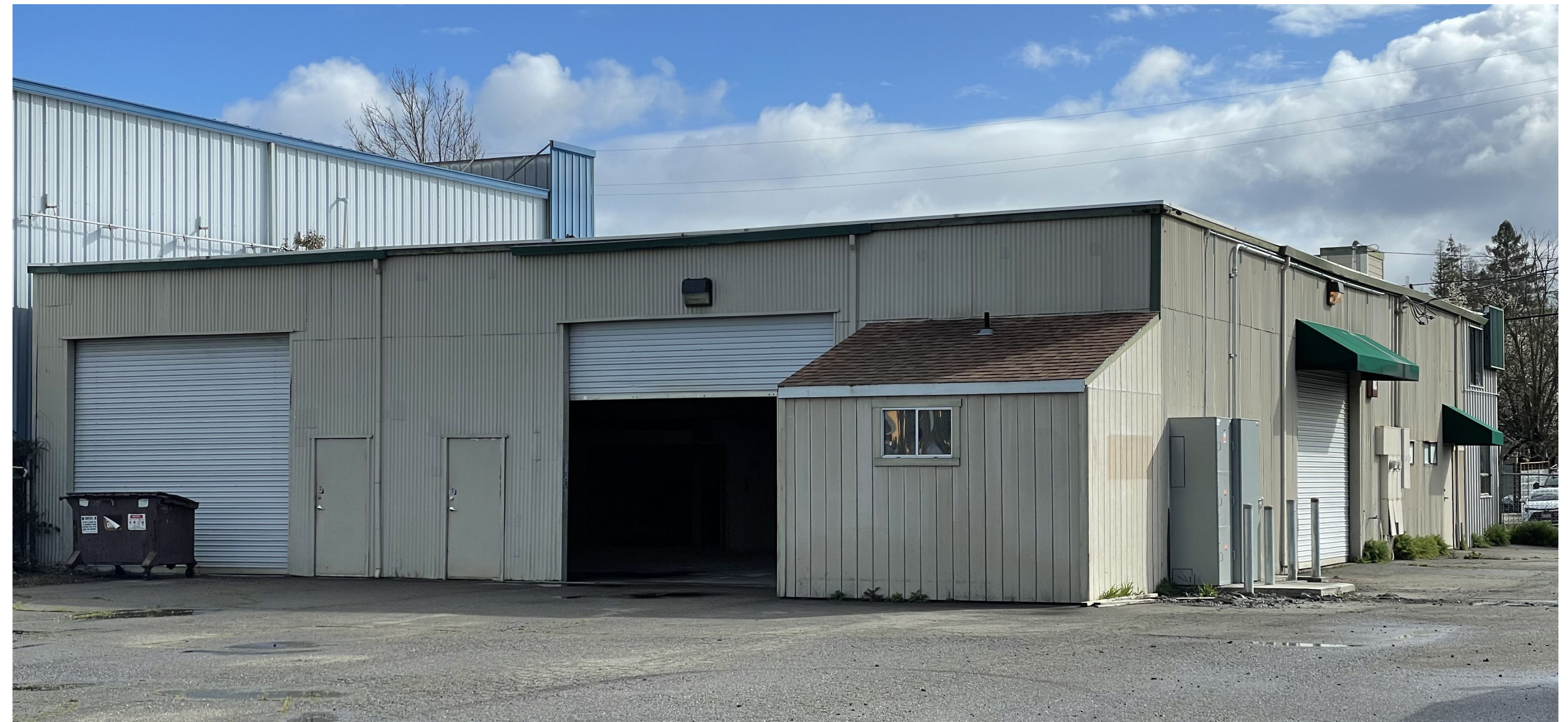
VIEW FROM SOUTH WEST
