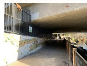
Existing metal fence along Greenway at 101 overpass. Height varies and pickets extend above top rail
