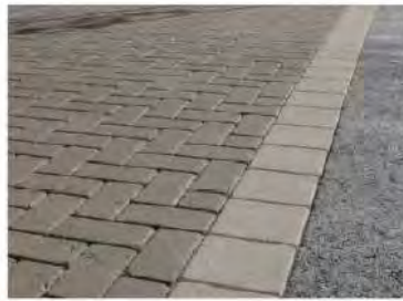
STAMPED ASPHALT AT PEDESTRIAN CROSSINGS
