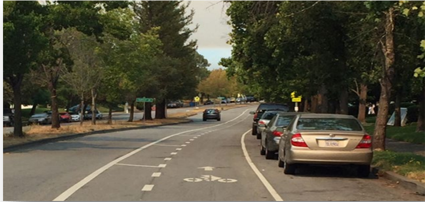
Where feasible the City has been adding a painted “buffer zone” to bike lanes to increase separation between cyclists and vehicle traffic. Buffer zone pictured here on West Third Street
