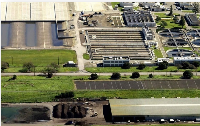
Laguna Treatment Plant biosolids program location
