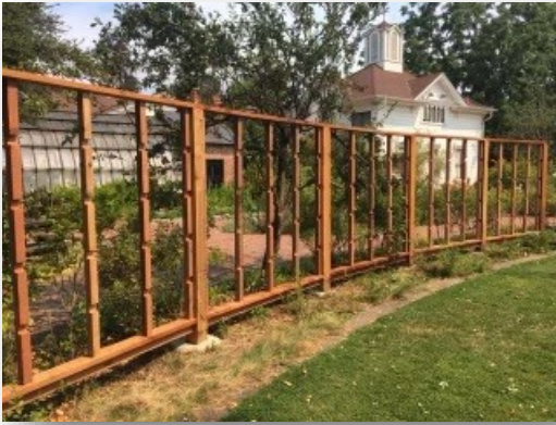
Luther Burbank Home and Gardens trellis fencing
