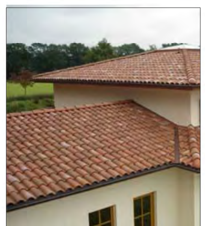
14 CONCRETE ROOF TILES
