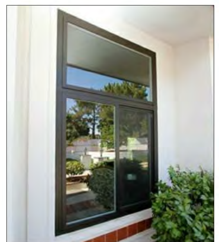
6 VINYL WINDOW SYSTEM - DARK BRONZE WITH CLEAR GLAZING - ON COURTYARD FACING WINDOWS
