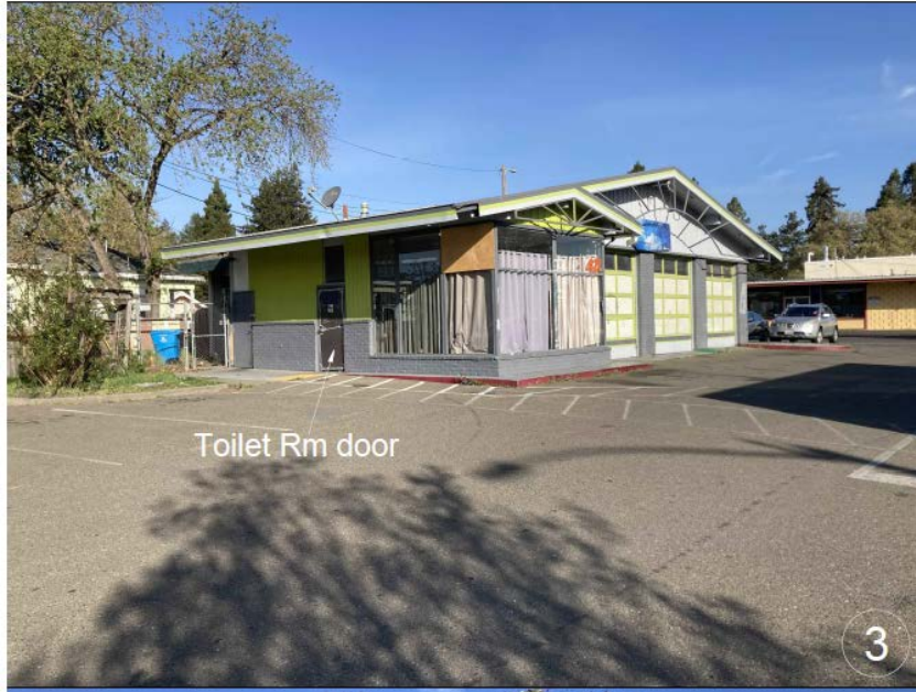
View of adjacent toilet room
