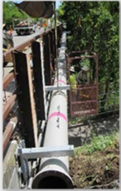
619 Miles of Water Main 28,824 Water Valves 23 Reservoirs
