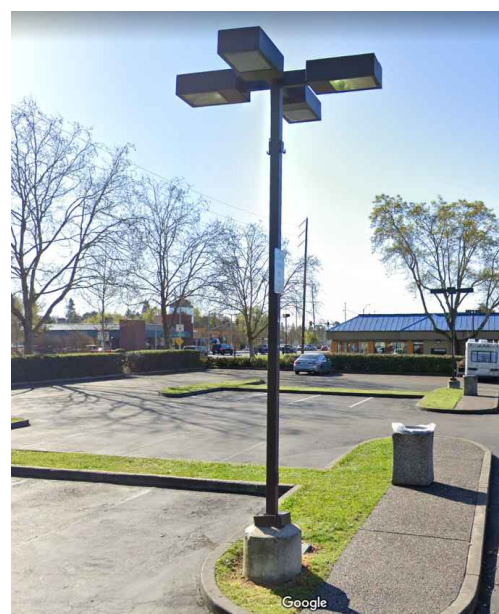
EXISTING LIGHT POLES THROUGHOUT SHOPPING CENTER
