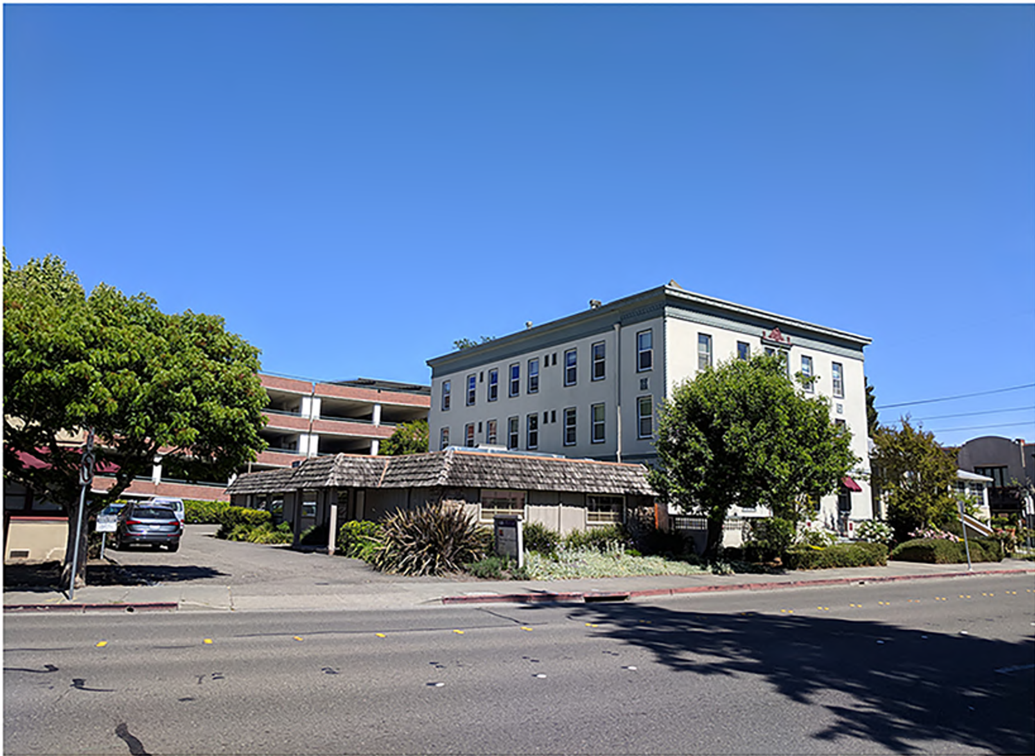
VIEW FROM B STREET
