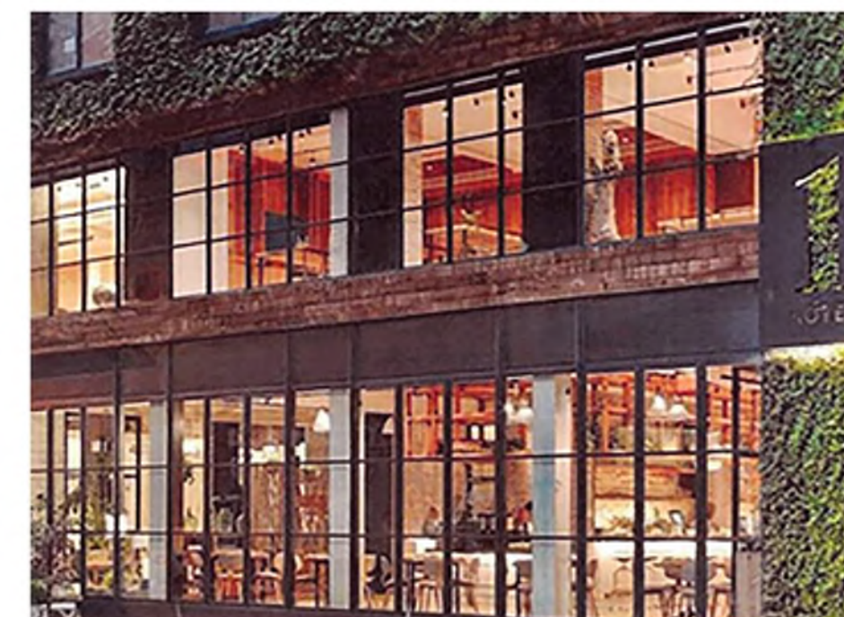
4 STEEL SASH STOREFRONT WINDOWS
