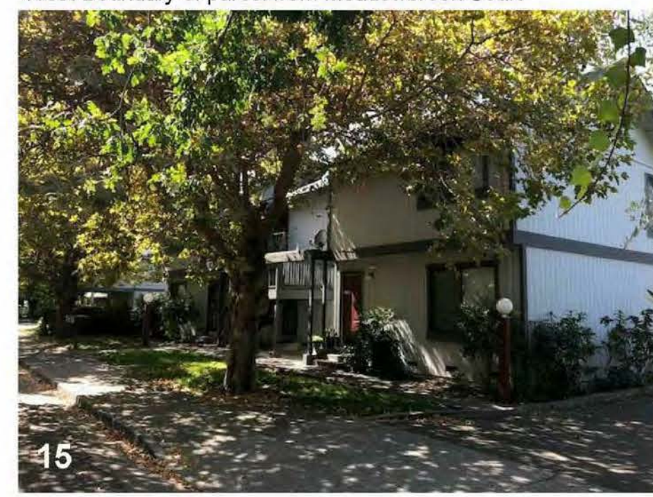
15 Apartment Buildings at west side of Meadowbrook Court
