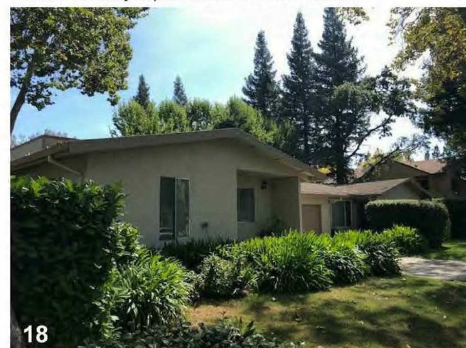
18 Single Family Residence at west side of Meadowbrook Court
