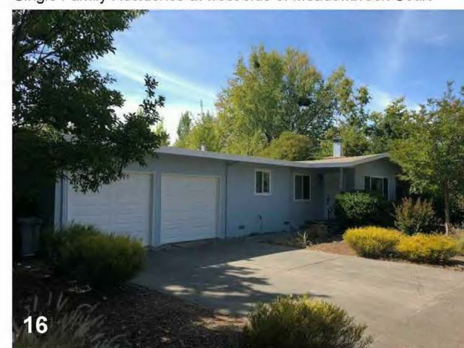
16 Single Family Residence at west side of Meadowbrook Court
