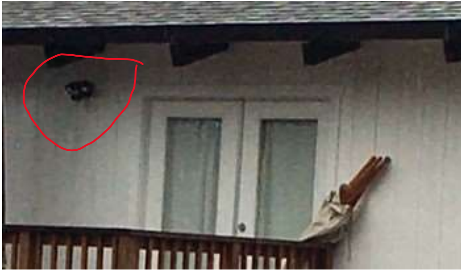
ACTUAL LOCATION OF LIGHT BETWEEN TWO SETS OF FRENCH DOORS (PHOTO FROM MARCH 2021)
