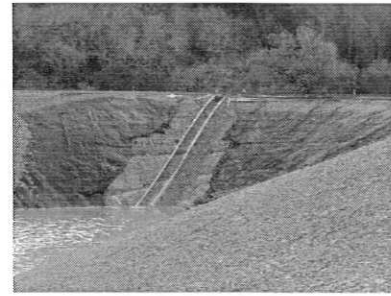
ALW Reservoir "D" During Construction
