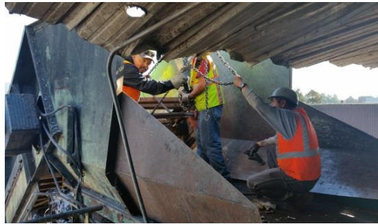
6) Repairing broken Infeed Conveyor – All sorting stopped
