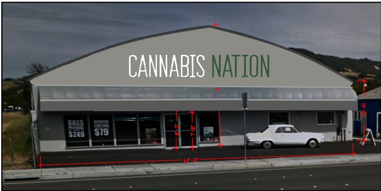
WEST / FRONT ELEVATION PHOTO
